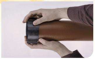
2. Push the EPDM rubber gasket over the end of the pipe or fitting, ensuring that the central inner register is abutted against the spigot end.
