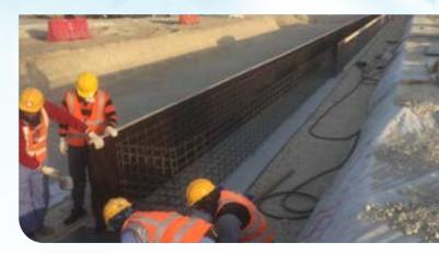
Fitting of the steel reinforcement cage can be carried out away from the trench, making the task easier for the contractor. The completed unit can then be lifted into the trench.
