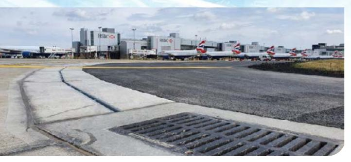
In some projects there may be a requirement to install the slot drain system to follow a given radius, for example around the perimeter of a taxi-way on an airport project, or following the curve of a landscape feature.
