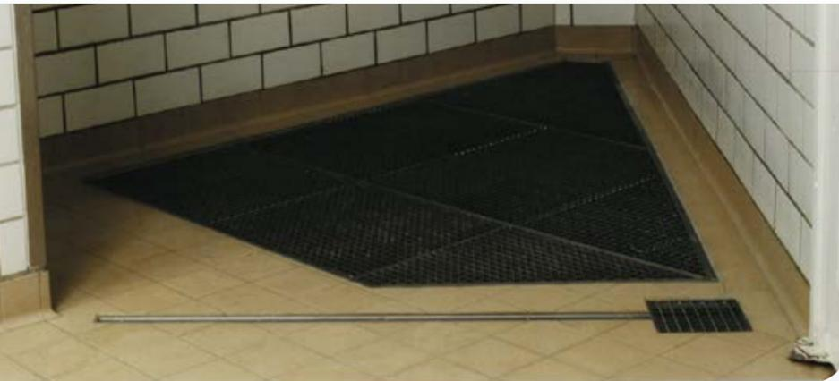
**Wash-down area gratings combined with Supaslot channel and integral stainless steel side inlet gully**
