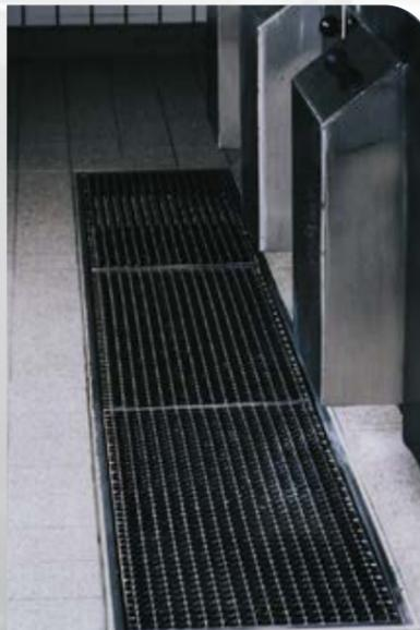
**Double notched anti-slip mesh gratings of stainless steel in a tiled floor**
