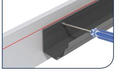
3) Using a string or laser to establish a true line and level of the gutter. Prepare to use packing pieces under gutter lengths where there are depressions in the fascia. Fix Gutters with No 12 x 38mm roundhead screws.
