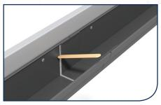
9) Tool-off displaced silicone sealant from the newly formed gutter joint. Allow to cure for 24 hours
