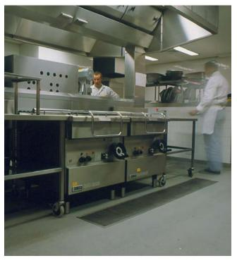
Heavy duty bar grating designed for trolley wheel-loading. Austenitic stainless steel channel and grating meet the high standards of hygiene demanded in today's working environments.
