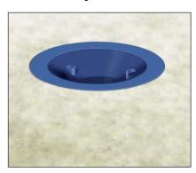
Install body such that flange is flush or sub-flush with roof deck. Ensure body is fixed securely, either bonded or clamped to the deck if not cast-in.
